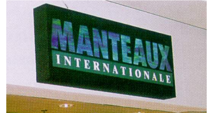
unacceptable - surface mounted box sign
