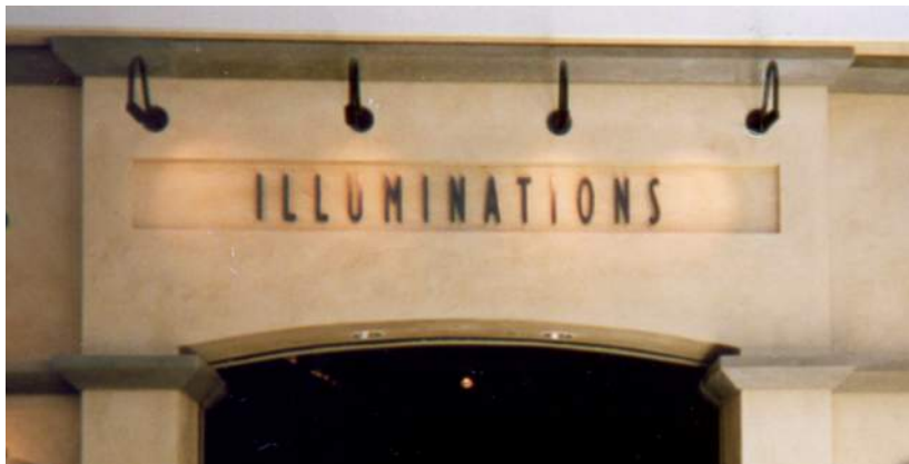
unacceptable - flat letters, illuminated with gooseneck lighting
