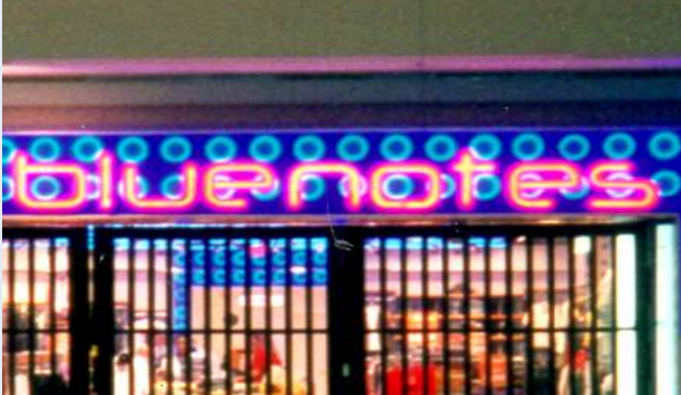
Exposed neon tube or open face channel letters with exposed neon tube.
