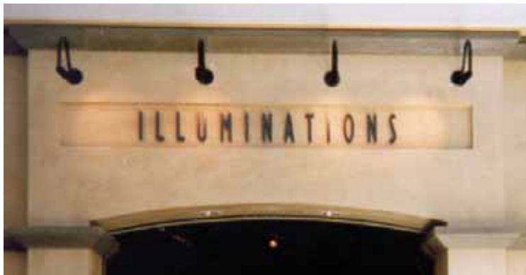
Unacceptable - flat letters, illuminated with gooseneck lighting
