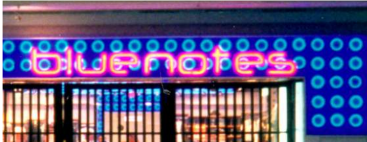
unacceptable - exposed neon tubes
