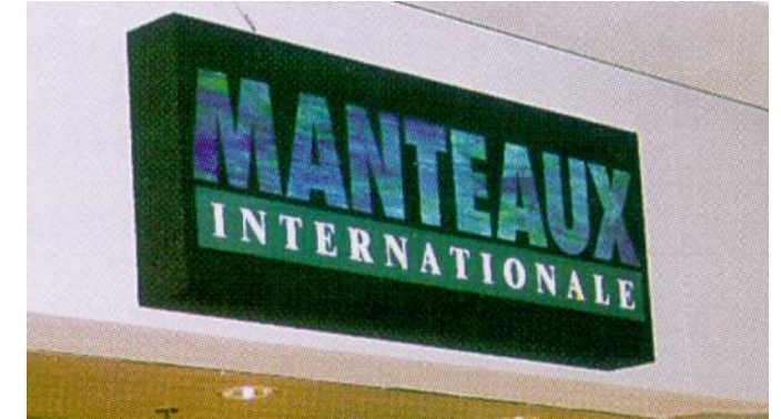
unacceptable - surface mounted box sign
