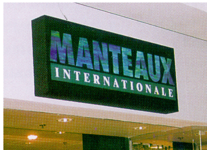
unacceptable - surface mounted box sign
