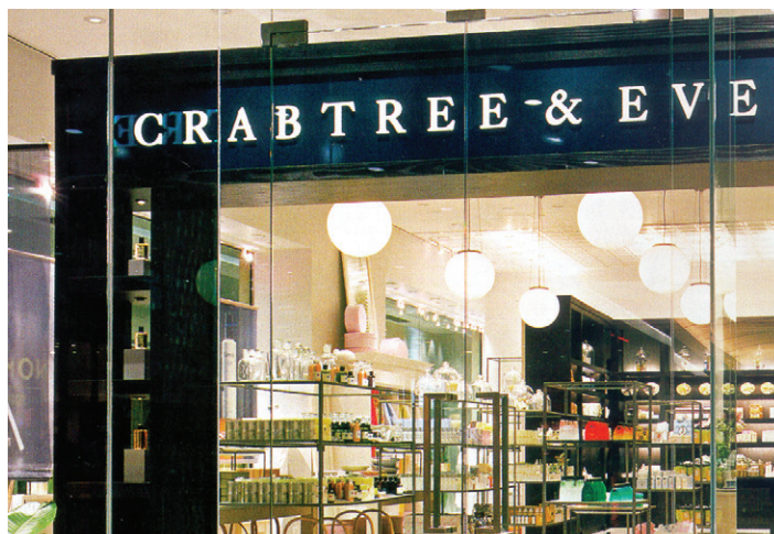
acceptable primary sign - internally illuminated push-through acrylic letters
