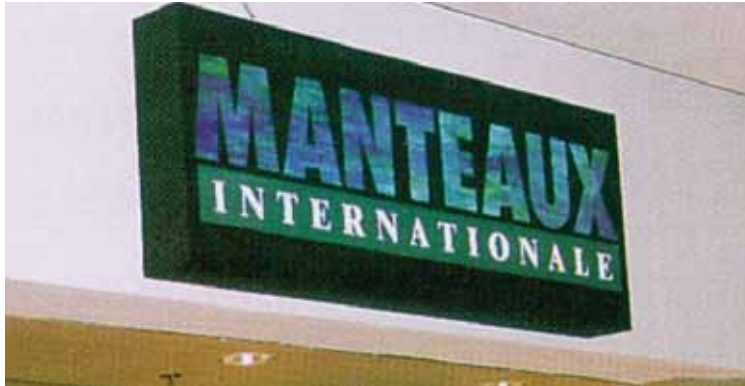
Unacceptable - surface mounted box sign
